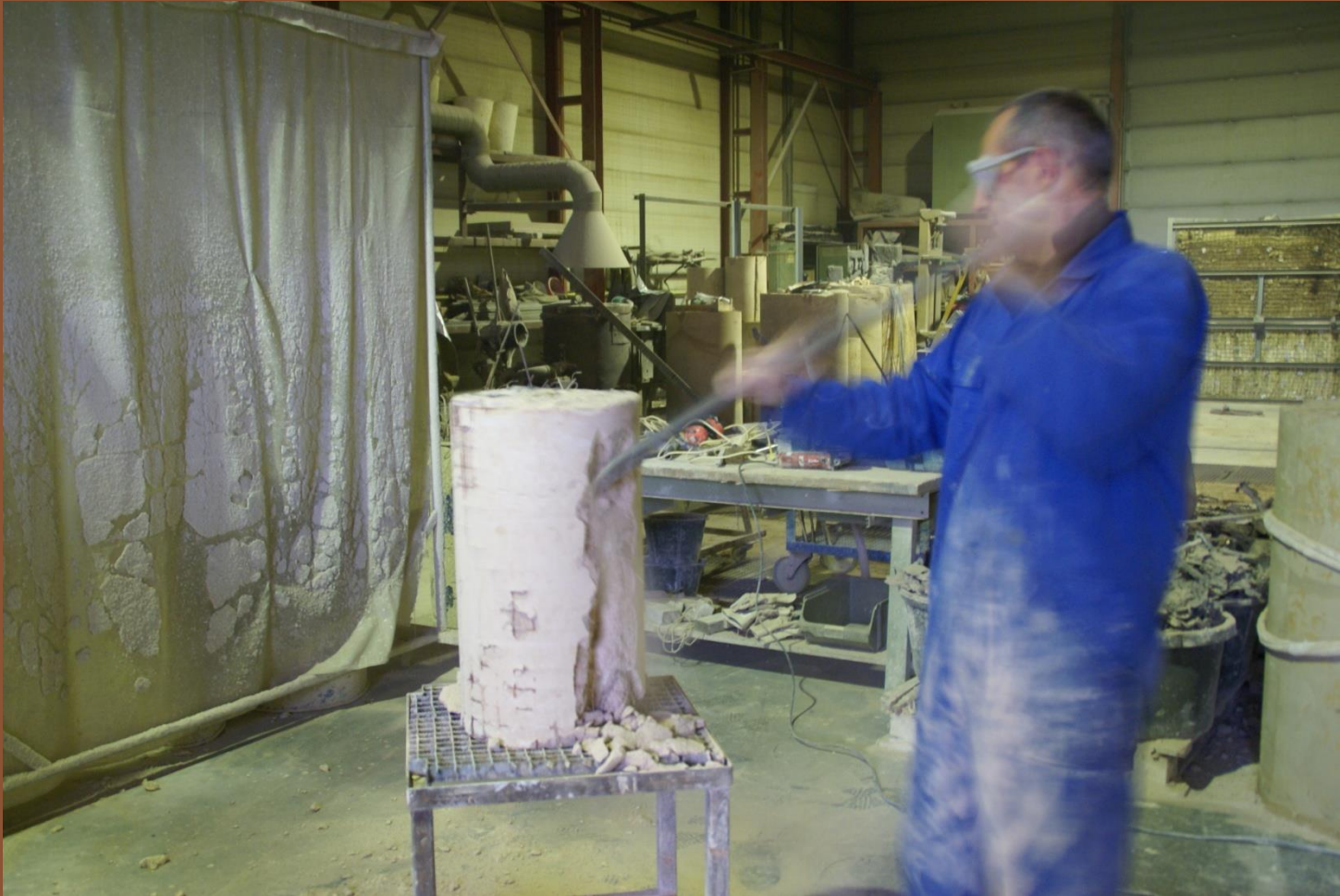
Removing the fireproof plaster
