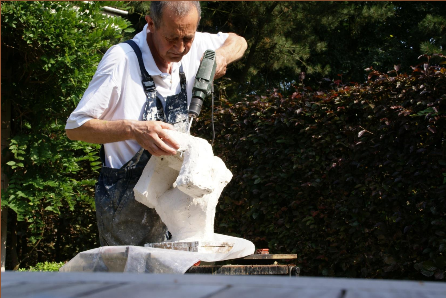
Preparing the connecting holes
